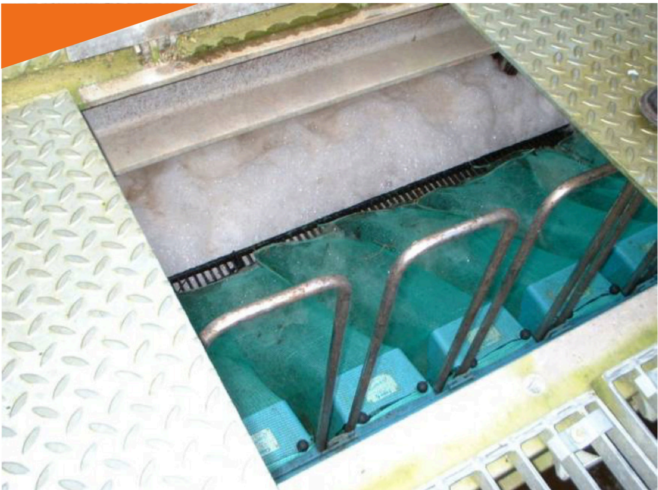
Figure 2: Surface water: 6 mm pre screening
