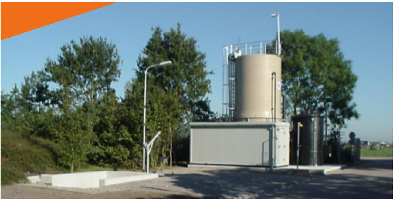
Figure 1 – WwTW Kaatsheuvel tertiary moving bed filtration.
