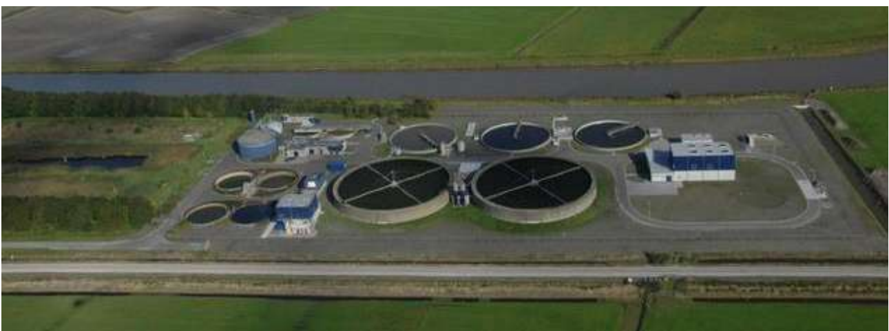
Figure 2 – Birdseye view of WwTW Franeker (site 1) with the MBF plant on the right
