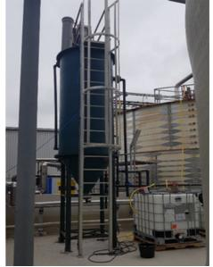
Figure 8 - Moving bed filter for solids removal
