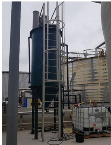
Figure 8 -Moving bed filter for solids removal
