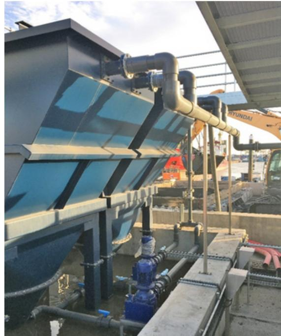
Figure 4 Tilted Plate Settlers being installed on site
